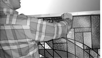
6. Install your permenant stops inside the frame for your Religious Image to set against. Place the stops as far away from the bulbs as possible to accomadate the image and the outside moulding. Next, place your image inside the frame. Drill a few ventilation holes in the top of the frame for air to escape.
