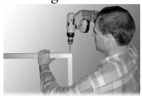
2. Construct your frame for your image, using 2"x 8" boards and screw them together. Before going any further, make sure you have left enough room for the image to be placed inside the frame.
